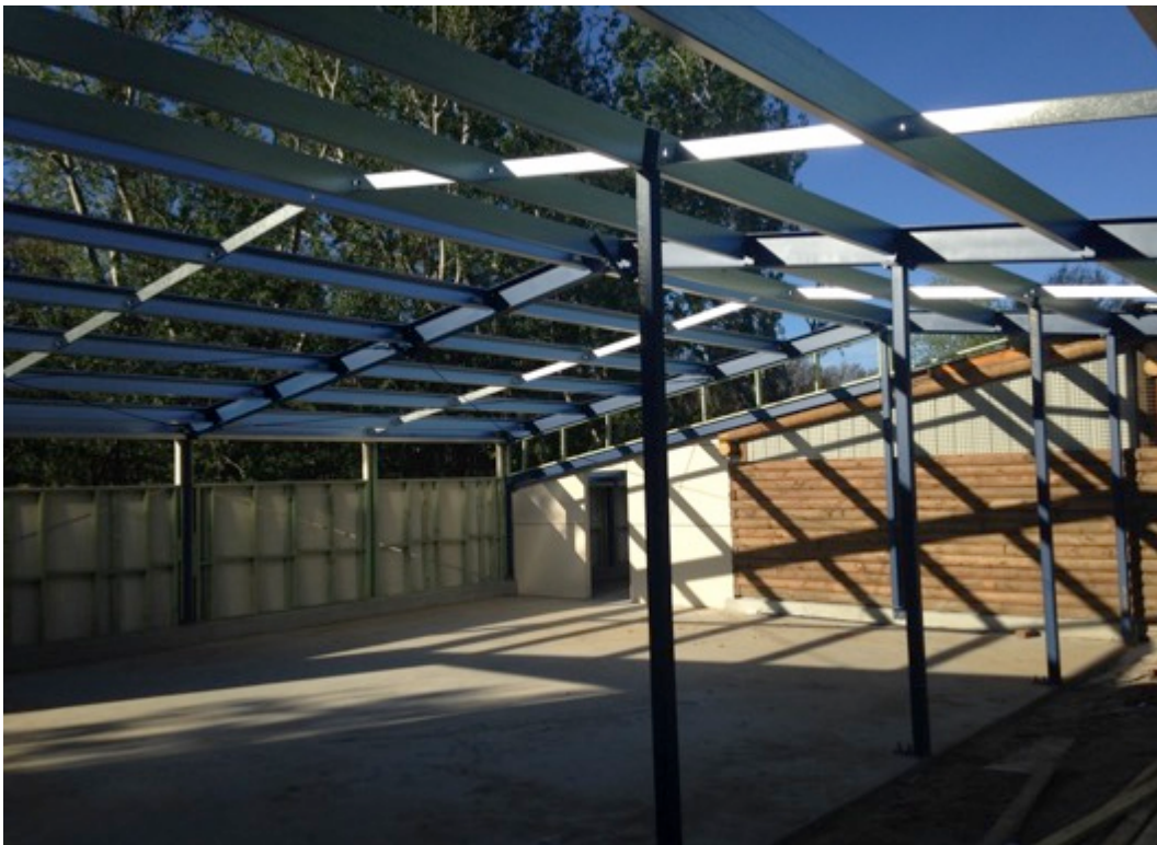
With walls as of 17 October
