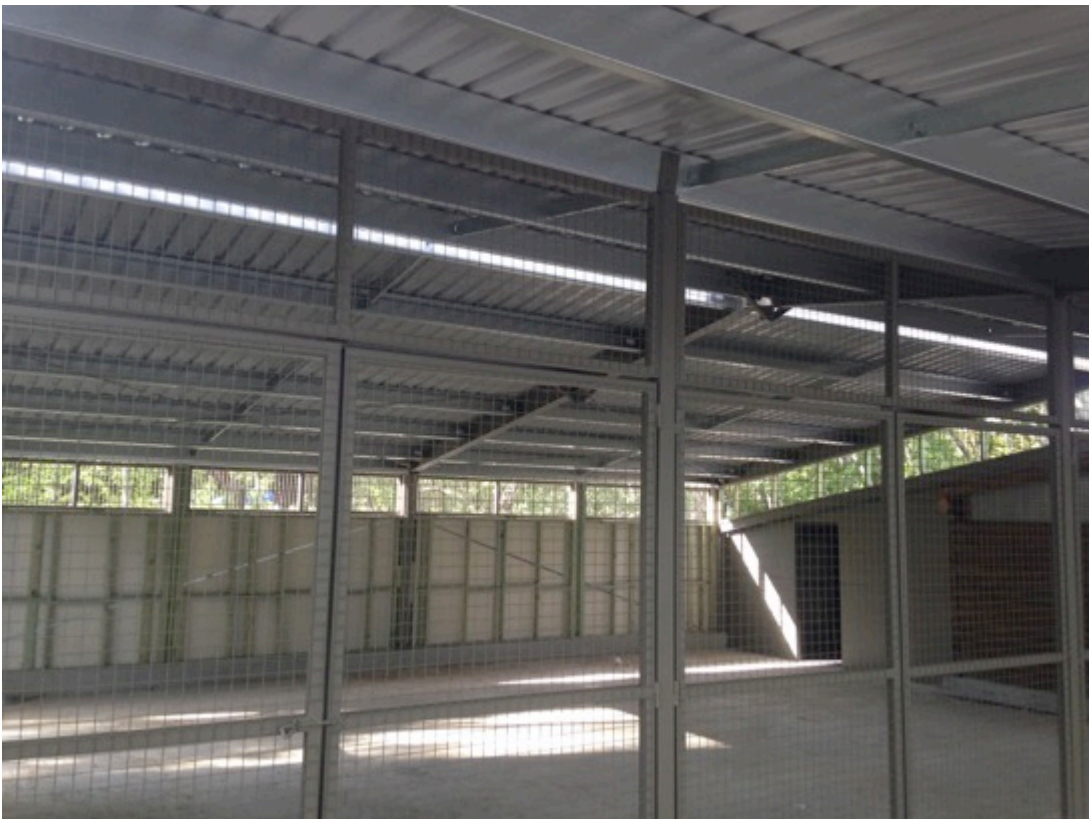
And with a roof as of 1 November
