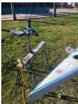
Drying the foam and glass in the damaged area on a Canberra winter's day – a bit of sun and a heat gun.
