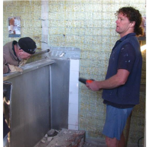
Right: Shane Lund supervising and Left: finishing off; the demolition of walls and troughs.
